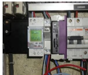
Installation also includes CityLone's driving system, comprised of one astronomical clock, one driving controller placed in the cabinet, one remote controller as well as SL31-EDA-ECS-P modules in each pole. This installation
