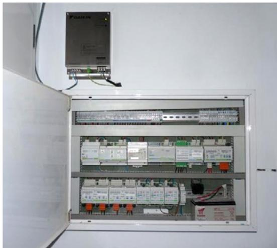
More than 2,000 controllers are installed throughout the property, making it one of the biggest residential automation projects using LonWorks® technology in Spain. Inside each home, residents can intuitively manage their environments (i.e., heated floors, HVAC, access control) via a touchscreen keypad and from a touchscreen tablet.
